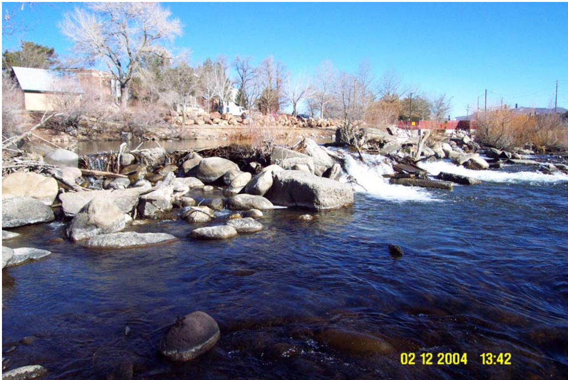
Figure 1. Existing Glendale Diversion
